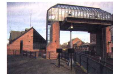
Foss Barrier and pump. Photo: carlos62/flickr CC.
